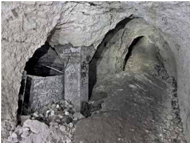
Beyond airshaft No.7 the tunnel has collapsed. Access to the tunnel beyond this point is accessible from another entrance. Note the water tank to the left. Photo Tim Wellburn
